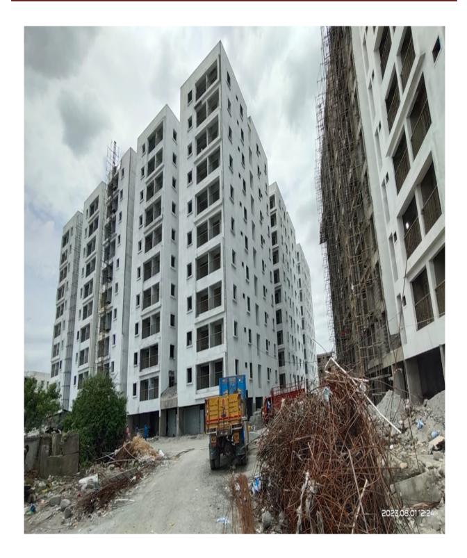
**Block D1:** External plastering overall 95% completed. 1<sup>st</sup> Coat Primer 95% completed. Internal Plumbing lines 90% & Sanitary Lines 35% completed.
