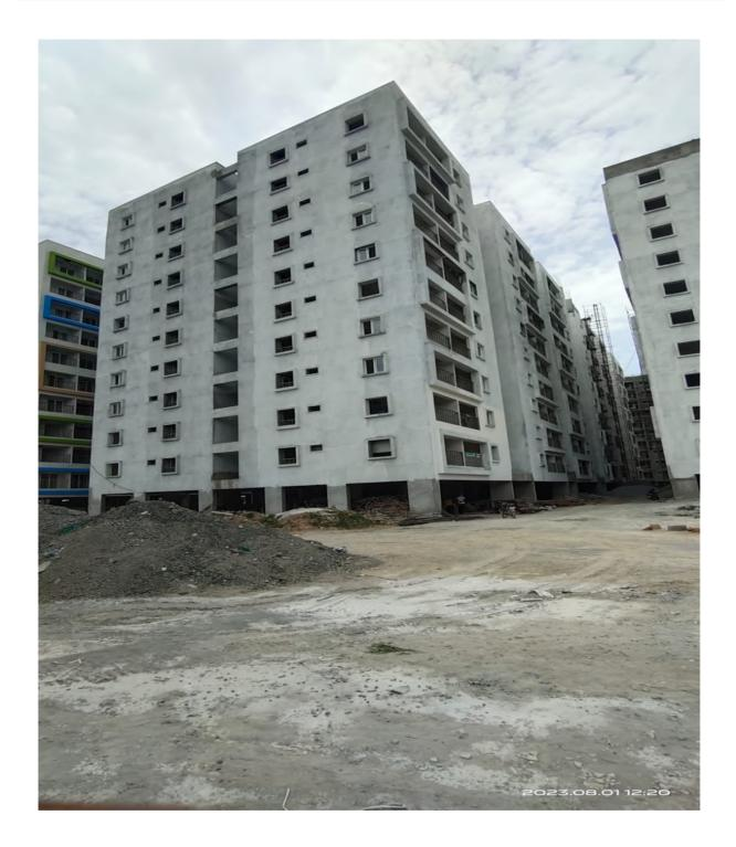
**Block C3:** External Plastering Overall 95% completed. 1<sup>st</sup> Coat Primer 95% completed. Internal Plumbing & Sanitary Lines 80% completed.
