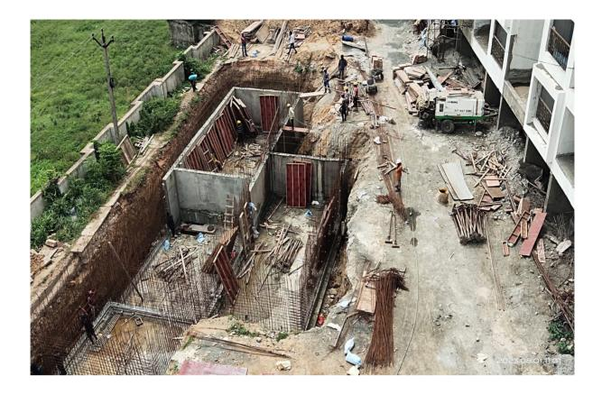
Underground Sump at B1-Block – P.C.C 100% completed.
